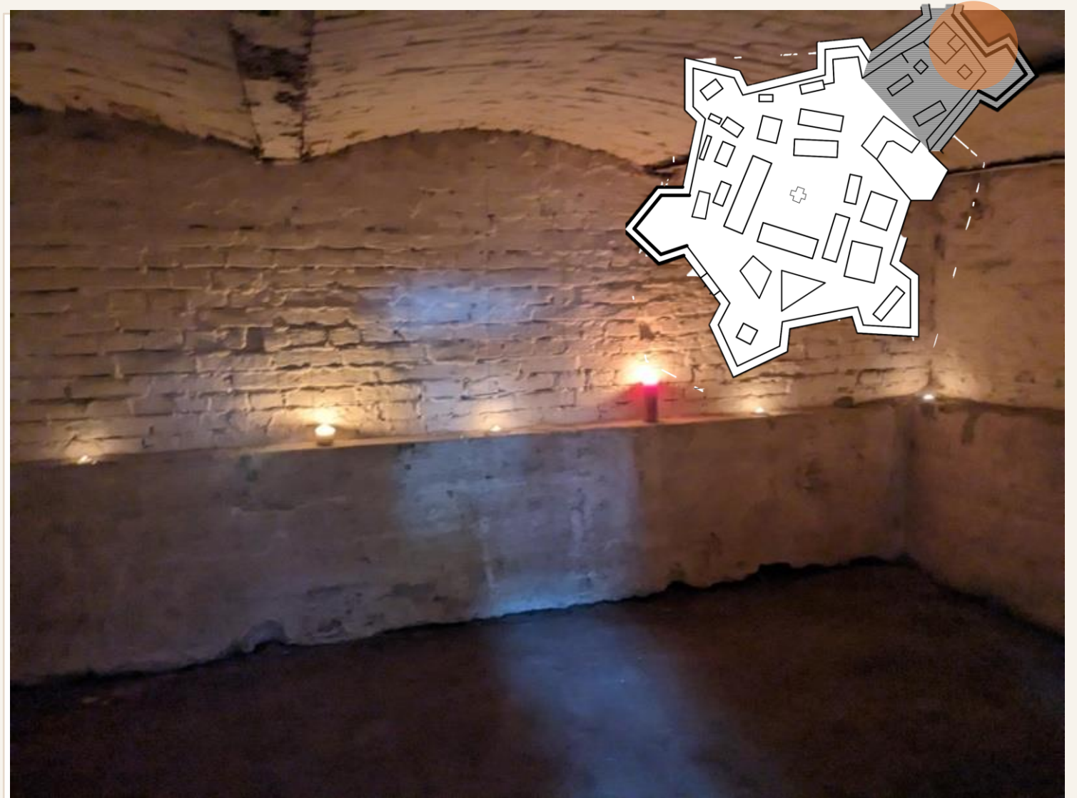
Restoration already changed the site
