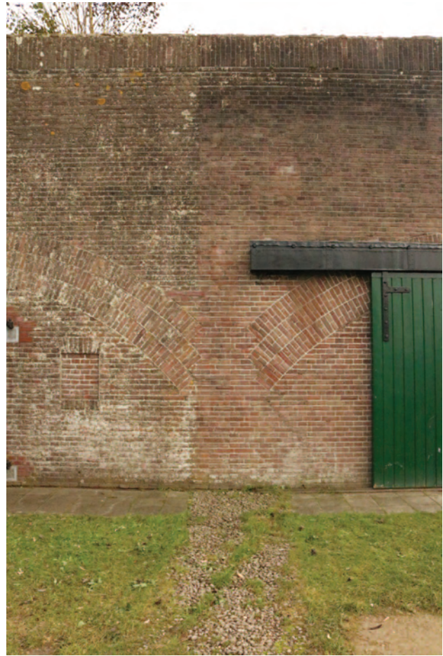
Figure 24 – Bunnik (NL), Fort bij Vechten, the bombproof barracks: partial cleaning of the façade in the portion falling within the strook (strip) (F. Marulo 2020).
