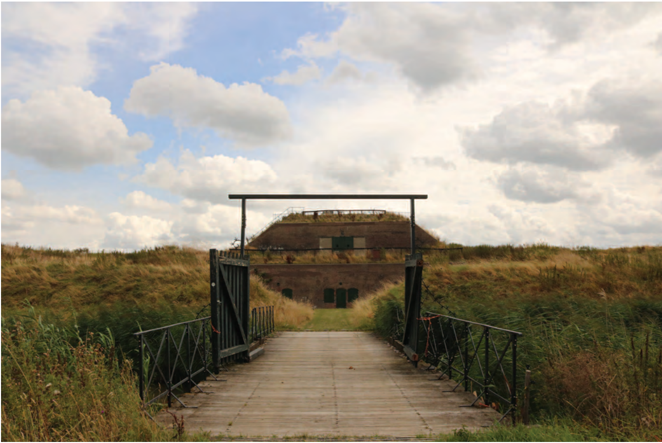
Figure 3 – Tull en 't Waal (NL), Werk aan de Waalse Wetering: the combination of synthetic (i.e., building) and natural components (i.e., water ditch, earthworks, camouflage vegetation) represent a distinctive feature of the forts of the New Dutch Waterline (F. Marulo 2019).
