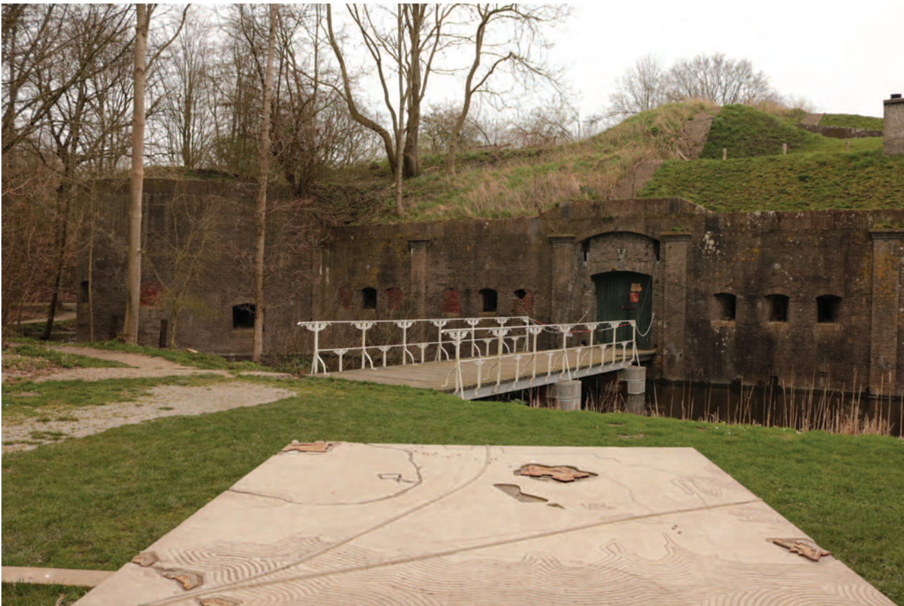
Figure 25 – Bunnik (NL), Fort bij Vechten, the central redoubt: exterior (front) after the intervention: earthworks and vegetation are restored to their 1880s layout only in that part of the building falling within the strook (strip) (F. Marulo 2020).
