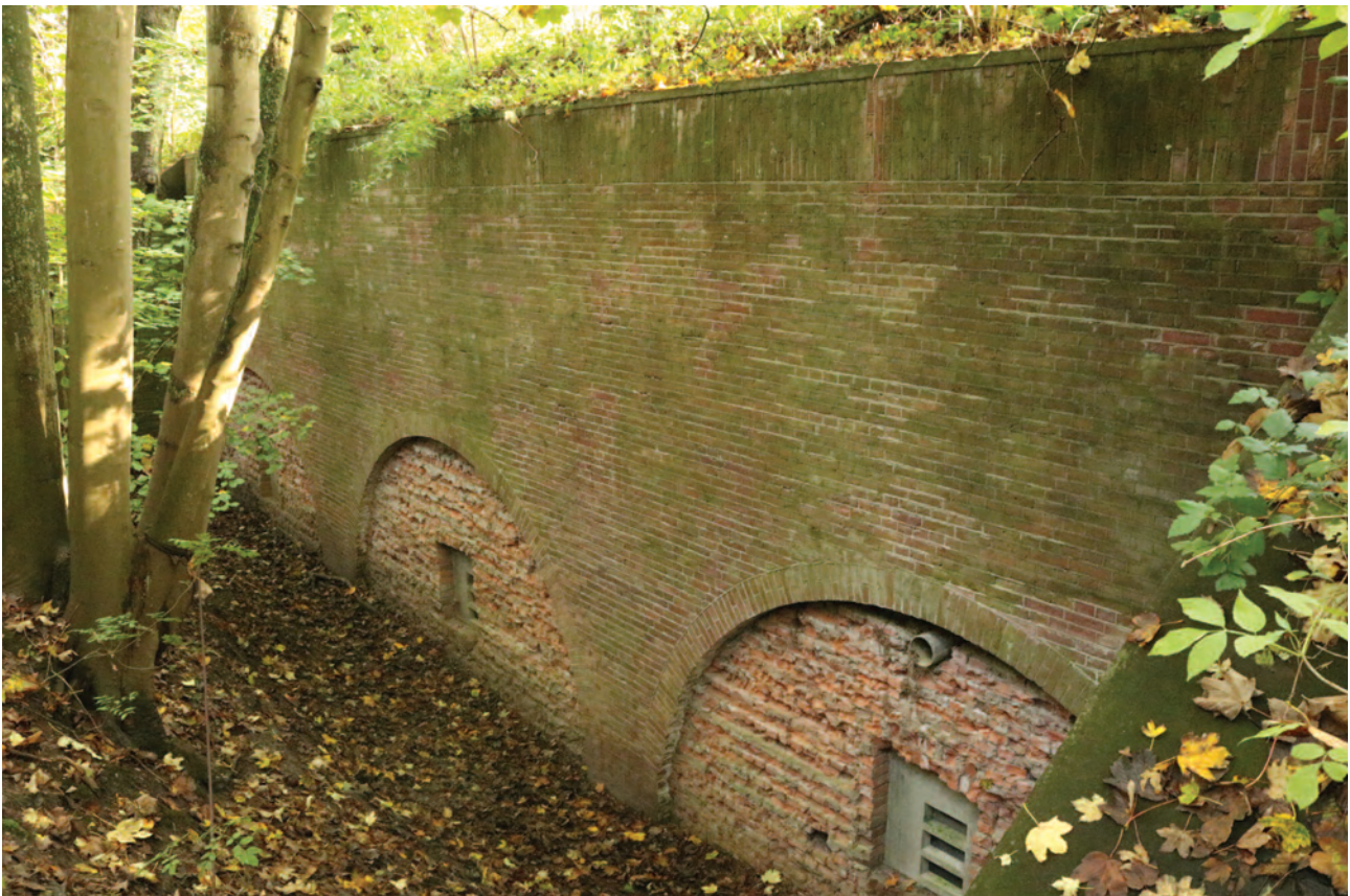
Figure 22 - Bunnik (NL), Fort bij Vechten: solution adopted to prevent (human) access to part of the buildings on the fort site for bat hibernation (design: BunkerQ) (F. Marulo 2020).
