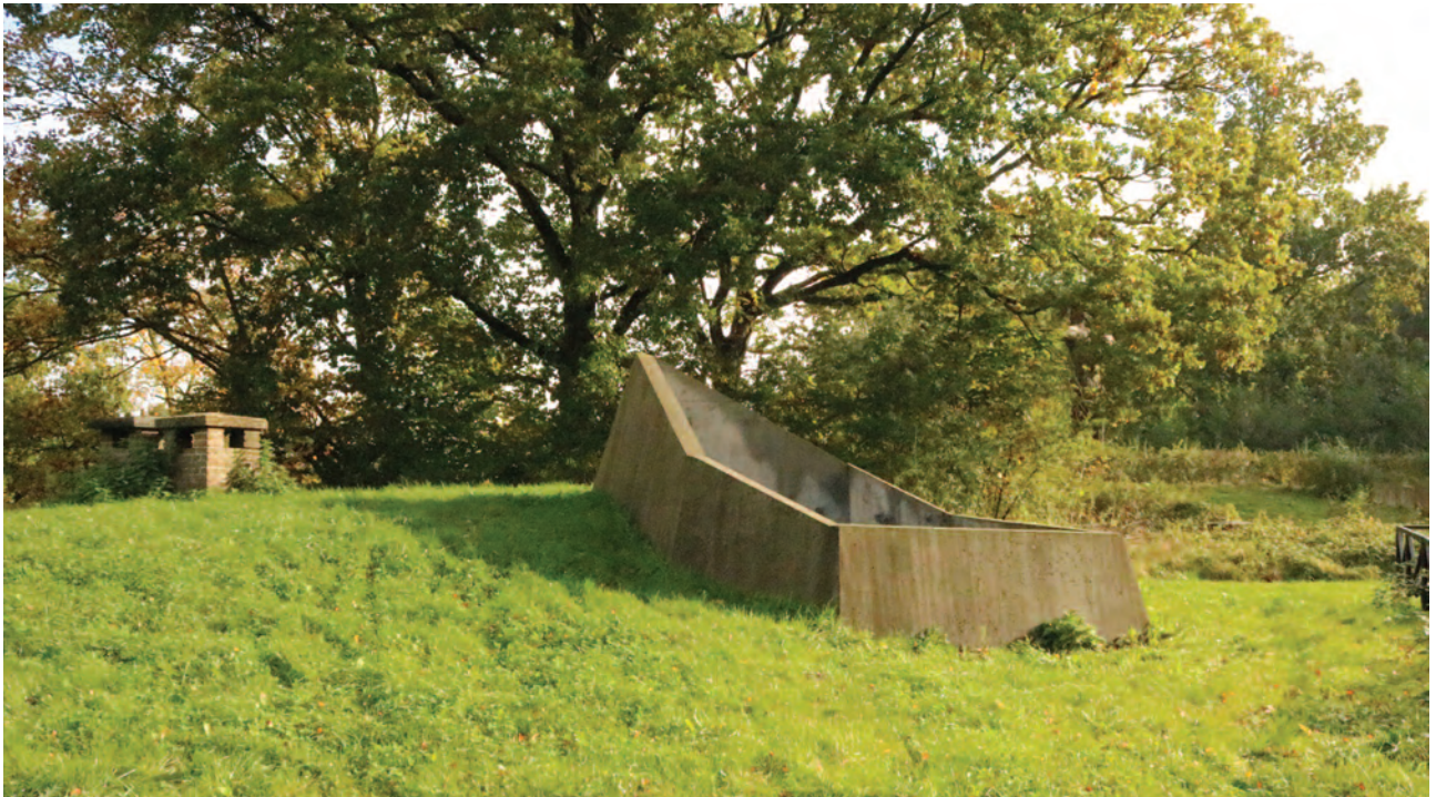
Figure 27 – Bunnik (NL), Fort bij Vechten, flank battery EL: the opening on the roof showing the functioning of the rain water collection system of the building (F. Marulo 2020).
