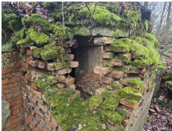
Fig. 5. Detached Brick Section and Moisture Saturated Area of the German Fortification
