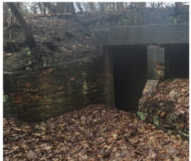
Fig. 5. Detached Brick Section and Moisture Saturated Area of the German Fortification
