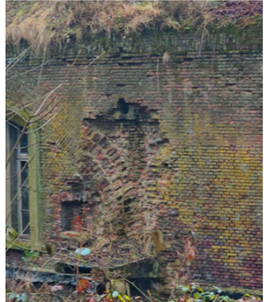
Fig. 4. Detached Brick Layers caused by the leaching of mortar from the wall
