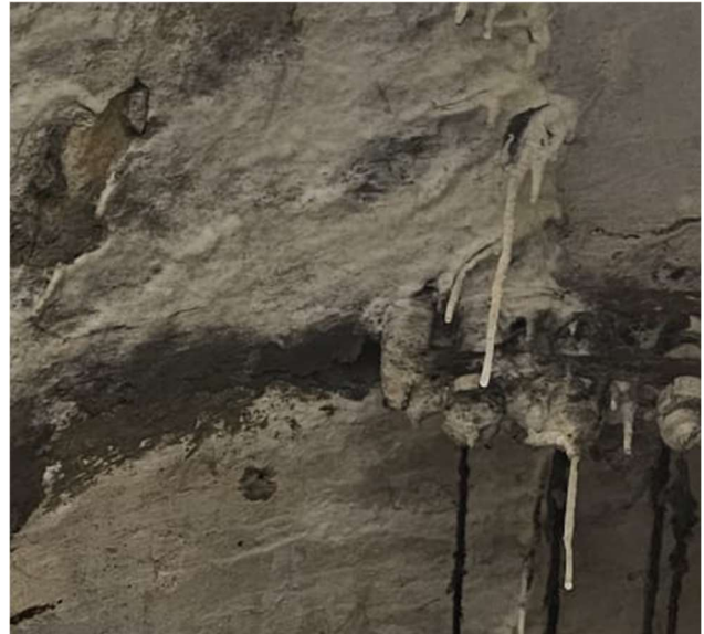
Fig.10. Salt deposition after re-crystallisation
