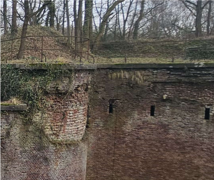
Fig. 4. Detached Brick Layers caused by the leaching of mortar from the wall
