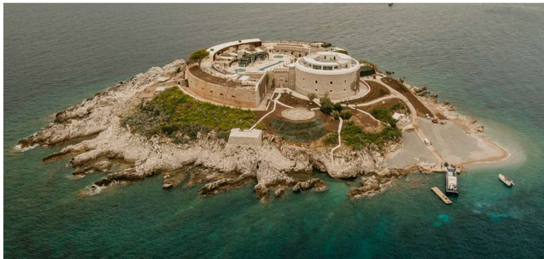
Images before and after the restoration Aerial view of the island
