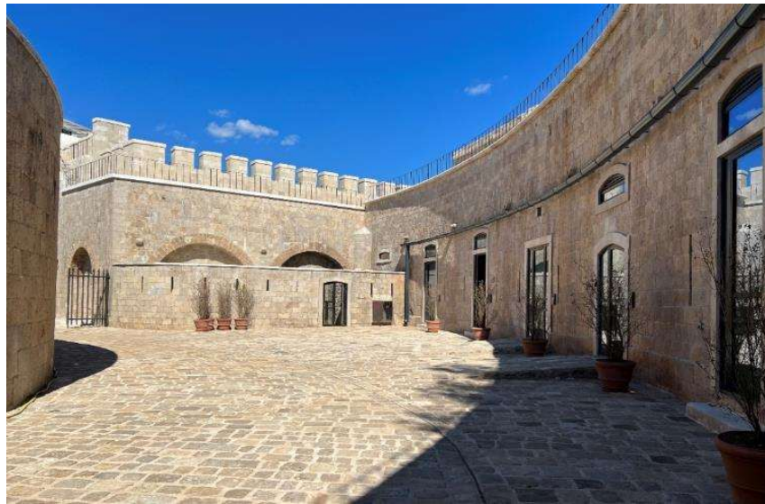
Images before and after the restoration The eastern lower courtyard with cannon rooms (casemates)
