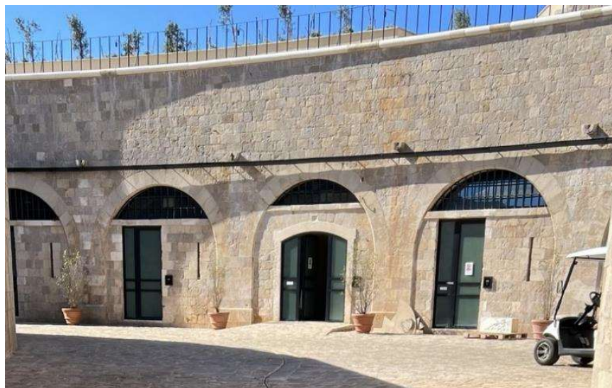
Images before and after the restoration The western lower courtyard with cannon rooms (casemates)
