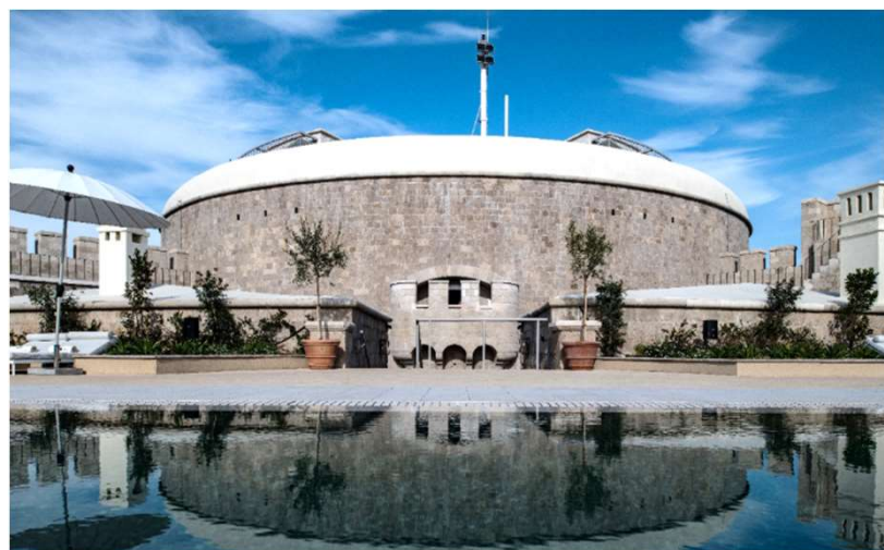
Images before and after the restoration Exerzierplatz (pool deck) and the tower
