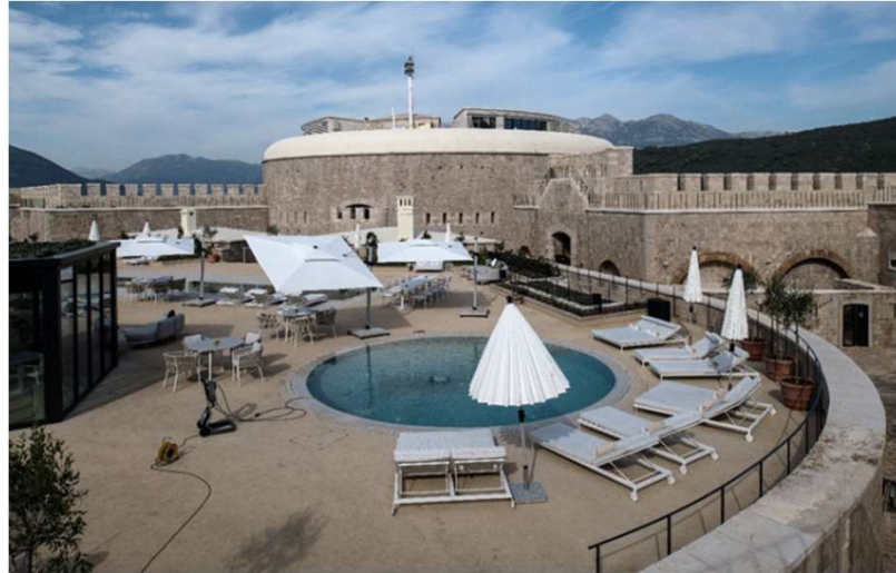
Images before and after the restoration Exerzierplatz (pool deck) and the tower
