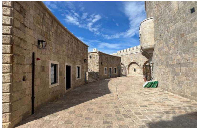
Images before and after the restoration Lower courtyard
